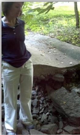
(2a) Stormwater Outfall Undermined by Channel Downcutting
