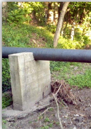
(2b) Sanitary Sewer Crossing – Concrete Pier Support Undergoing Scour
