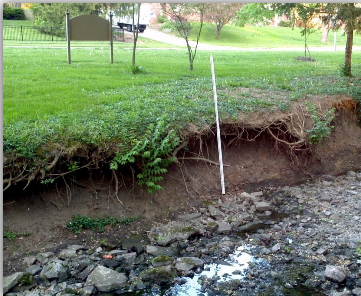
(1a) Active Bank Failure Downstream of the Pedestrian Bridge adjacent to Zandale Park Entrance Sign
