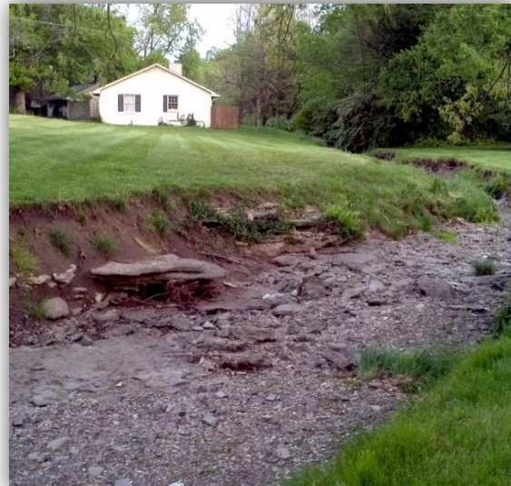
(5c) Looking Downstream from the Culvert Crossing at Lansdowne Estates—Note the Limestone Bedrock on the Channel Bed and Protruding from the Left Bank
