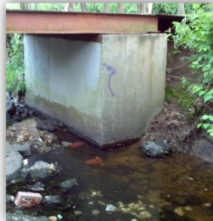
(2c) Pier Scour and Flanking of Pedestrian Bridge
